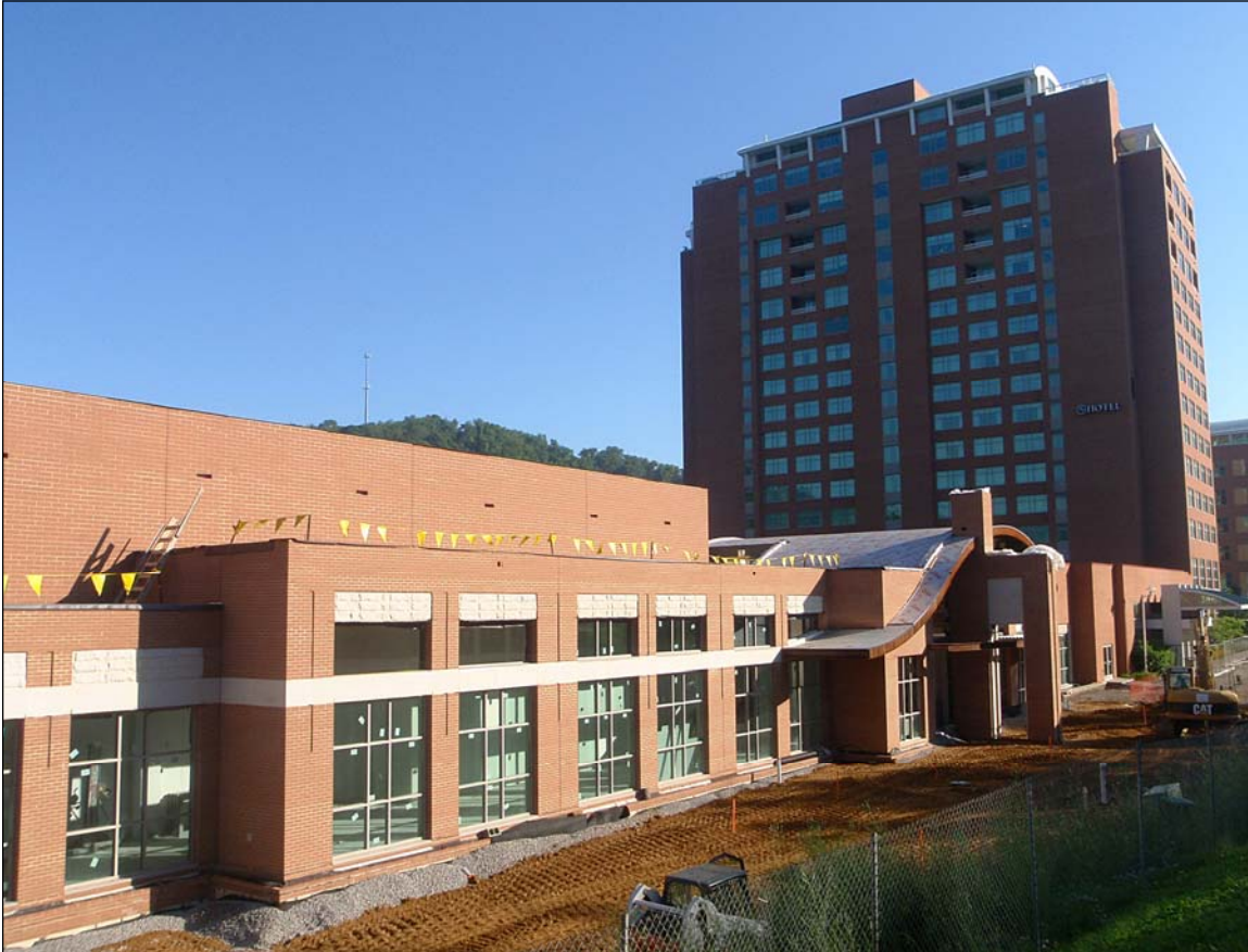
(Currently Under Construction)
